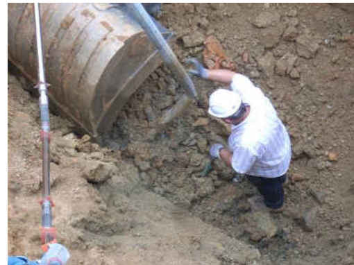
Fig. 9. Removal of D.M.S. column.
