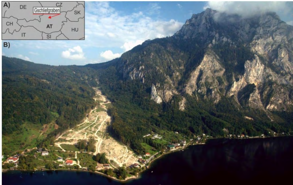
Fig. 1: General setting of the Gschliefgraben site: (A) Position within Austria, (B) Airborne photo of the Gschliefgraben valley and Mt. Traunstein from the west (Photo by: R. Supper, 2009).
