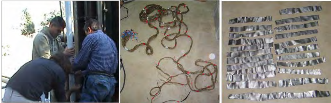
Fig. 2: (left) Installation of the multi-node cable on the outer surface of the plastic piezometer that was placed inside the borehole. (right) Custom made multi-node cable with 48 electrode outputs and lead leaves that were used as borehole electrodes.
